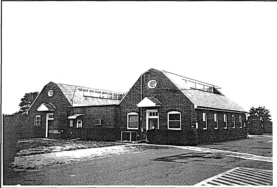
Photo ID: Building 1044 and 1045, North and East Facades, 4/97
