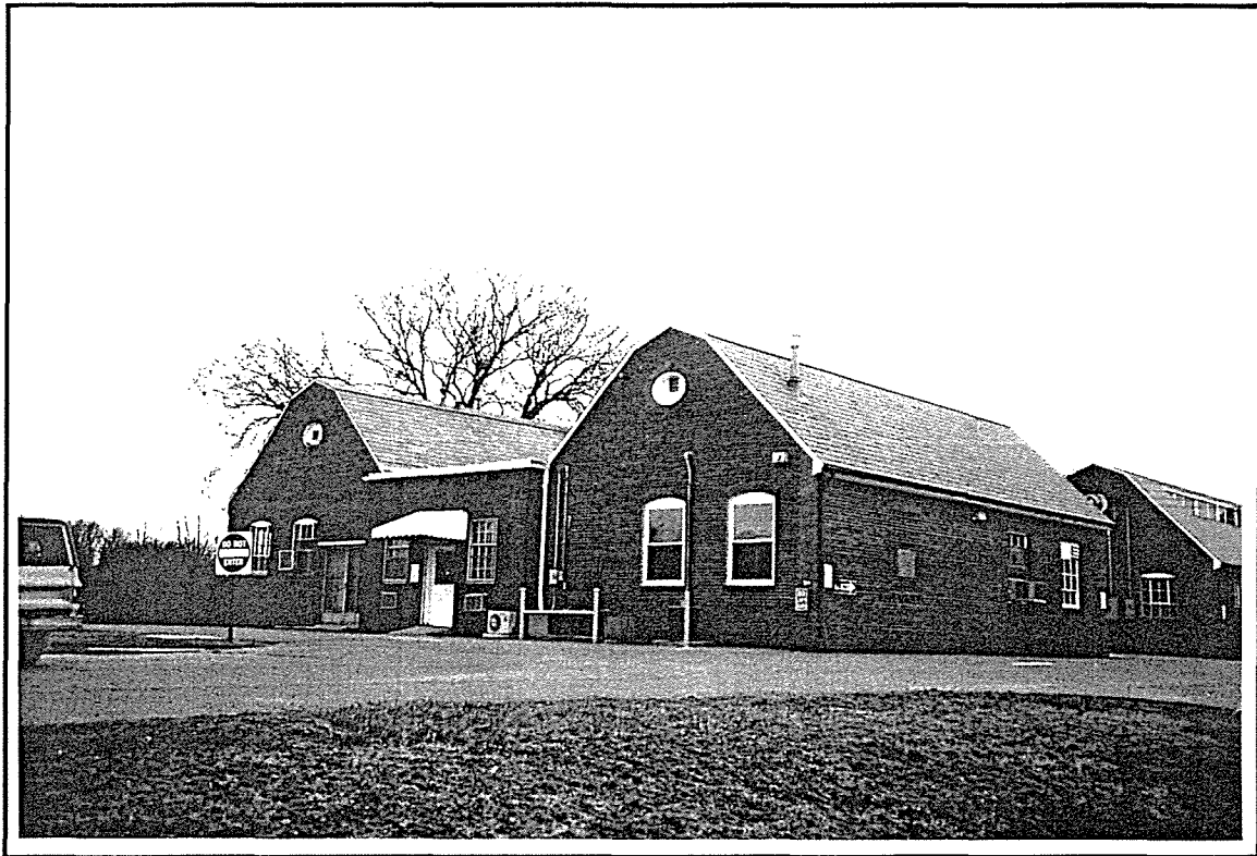
Photo ID: Building 1041 and 1042, North and East Facades, 4/97
