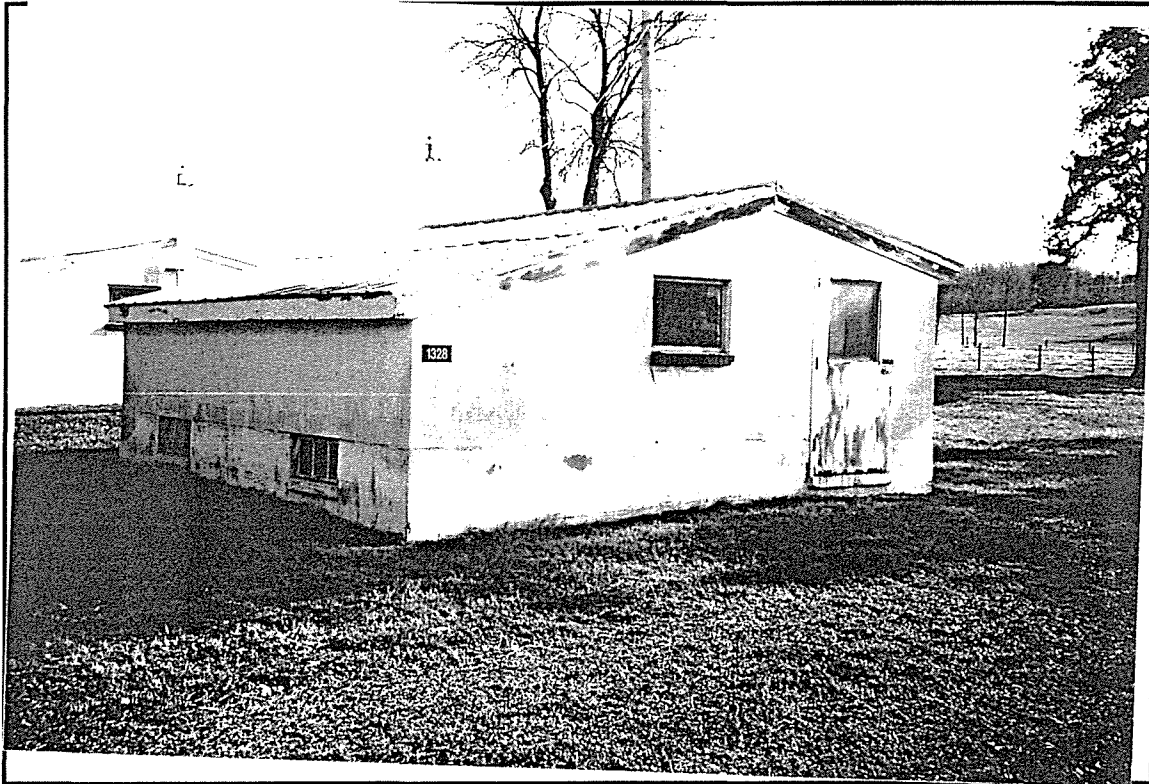
Photo ID: Building 1328, North and West Facades, 12/97
