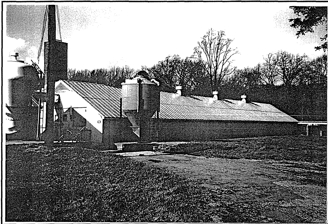
Photo ID: Building 1425, South and East Facades, 12/97
