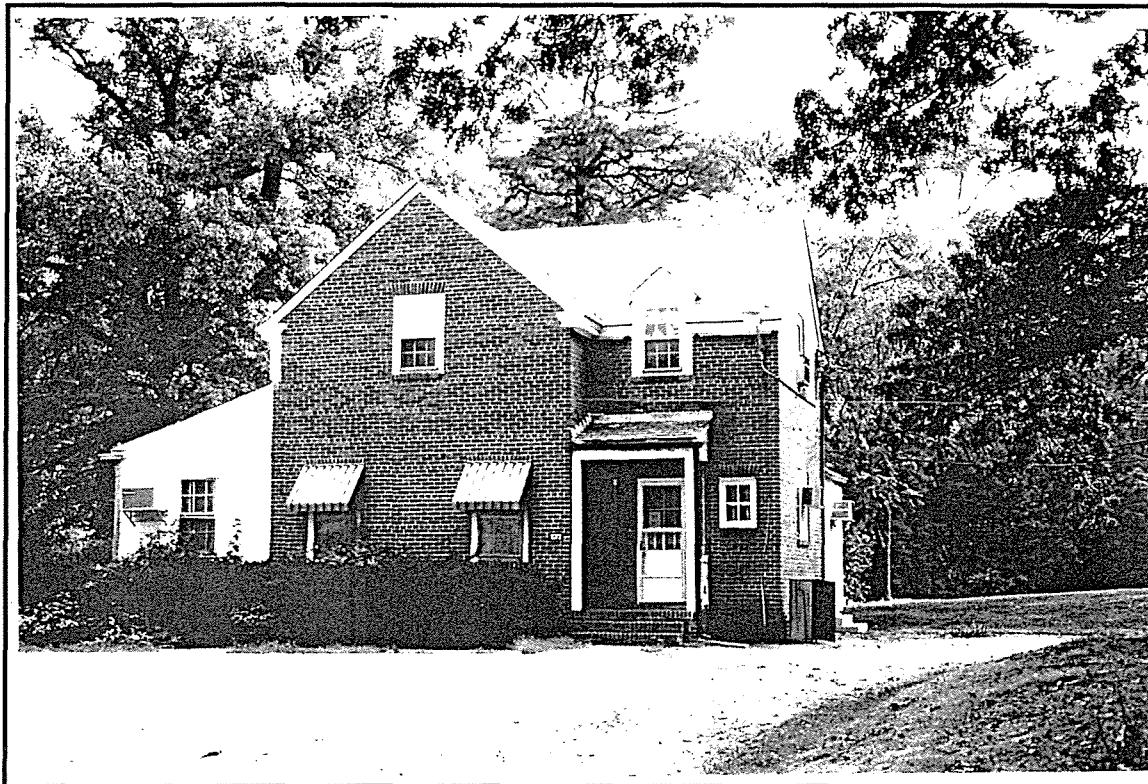
Photo ID: Building 1072, North and West Facades, 9/97
