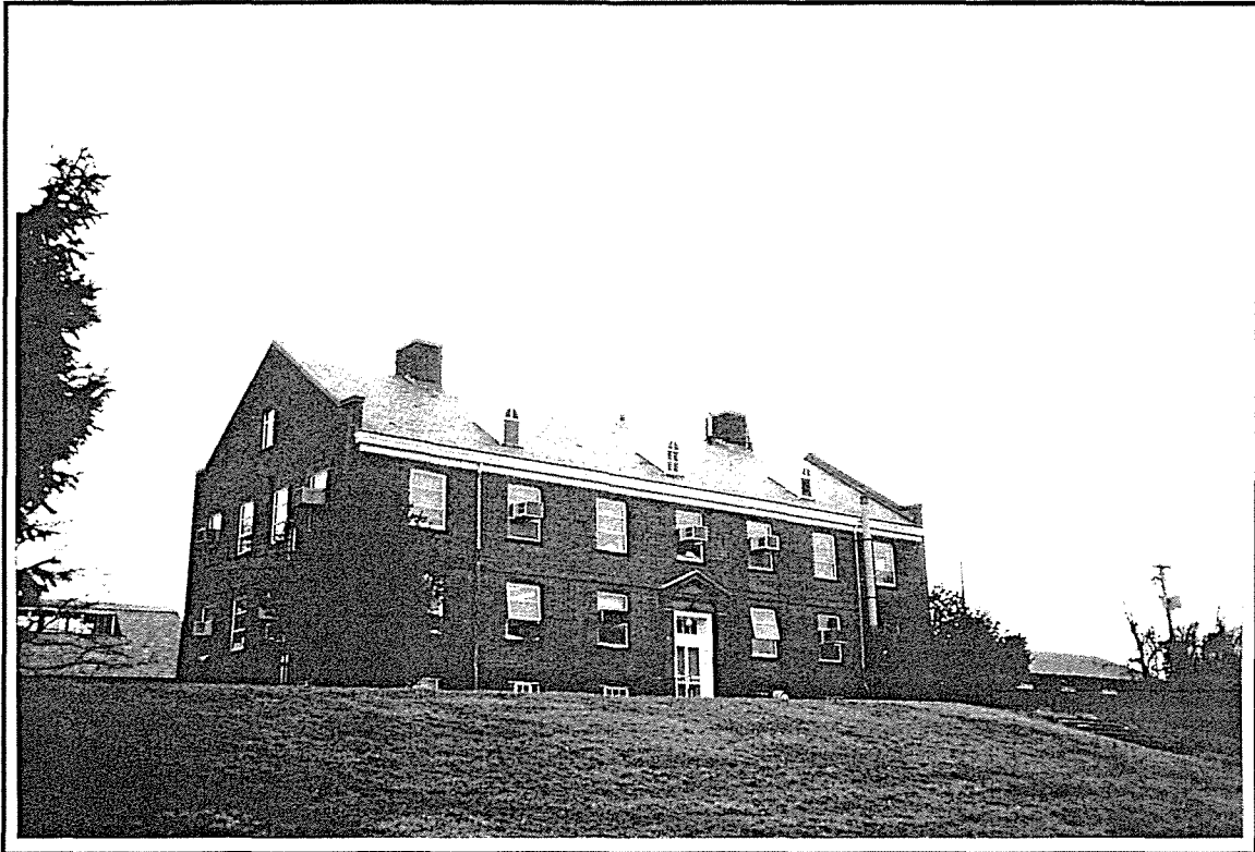
Photo ID: Building 1040, North and East Facades, 4/97
