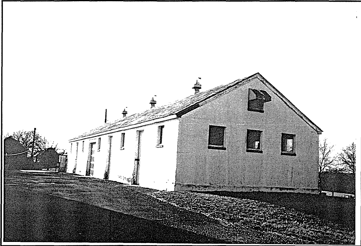
Photo ID: Building 1122, East and South Facades, 4/97
